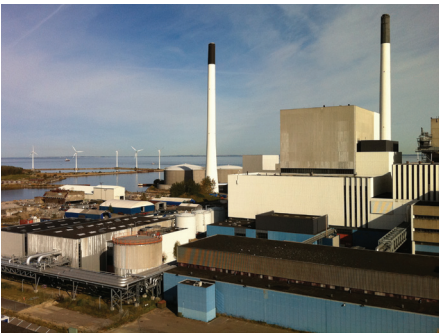
Waterfront view from roof of Amagerforbrænding.
